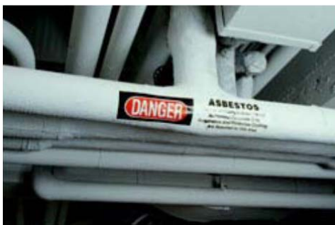
Good Practice: Asbestos-coated pipes are properly marked.
