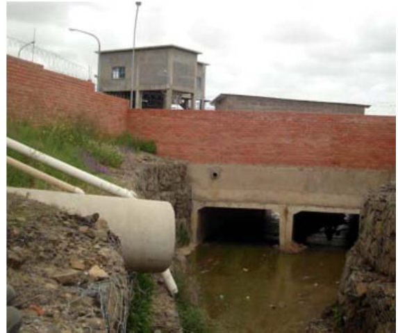
ZTV Bad Practice: Factory wastewater must not bypass wastewater treatment.
